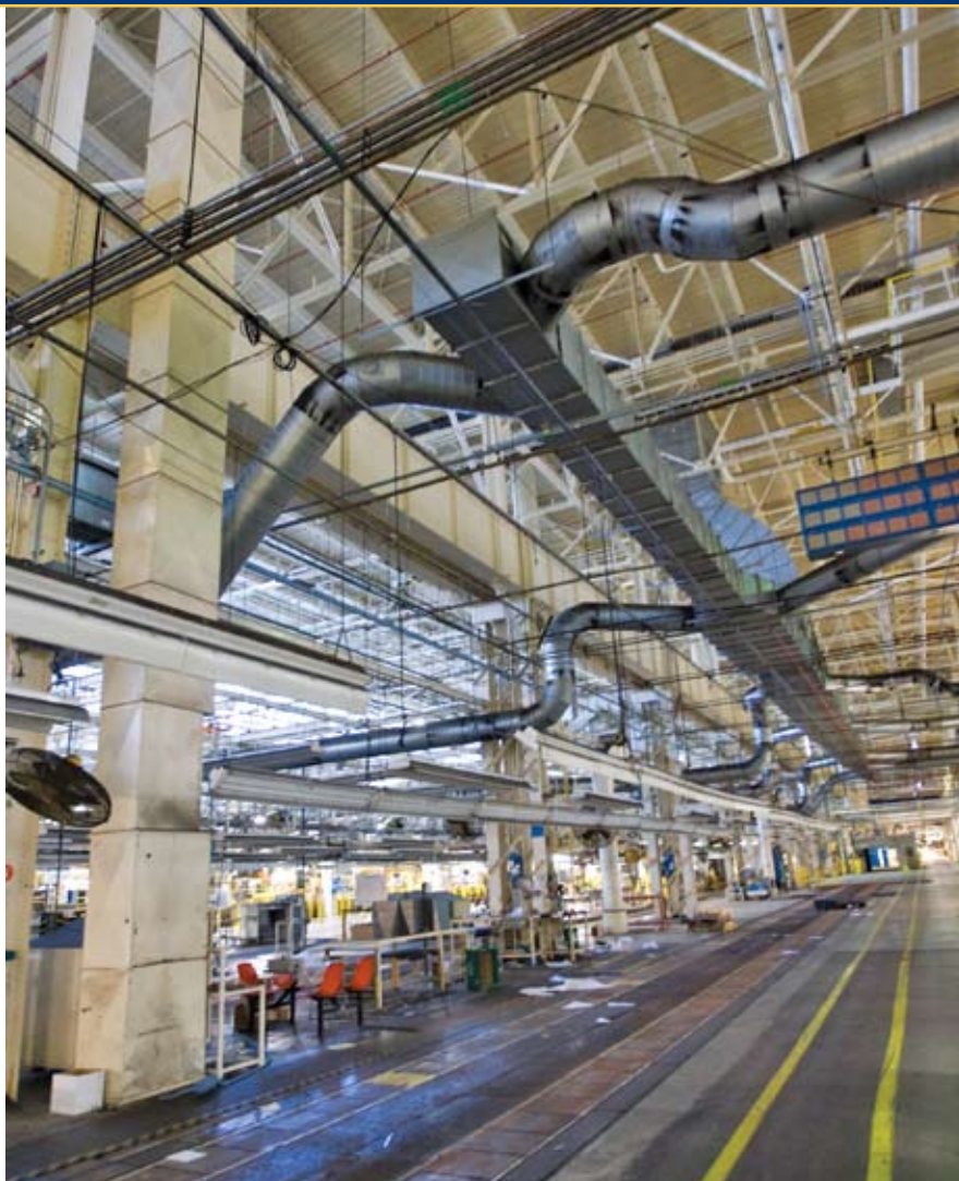
The former Chrysler automotive assembly plant in Newark was acquired by the University of Delaware late last year for about $24 million. The 272-acre site is being converted into a high-tech science and research campus.
