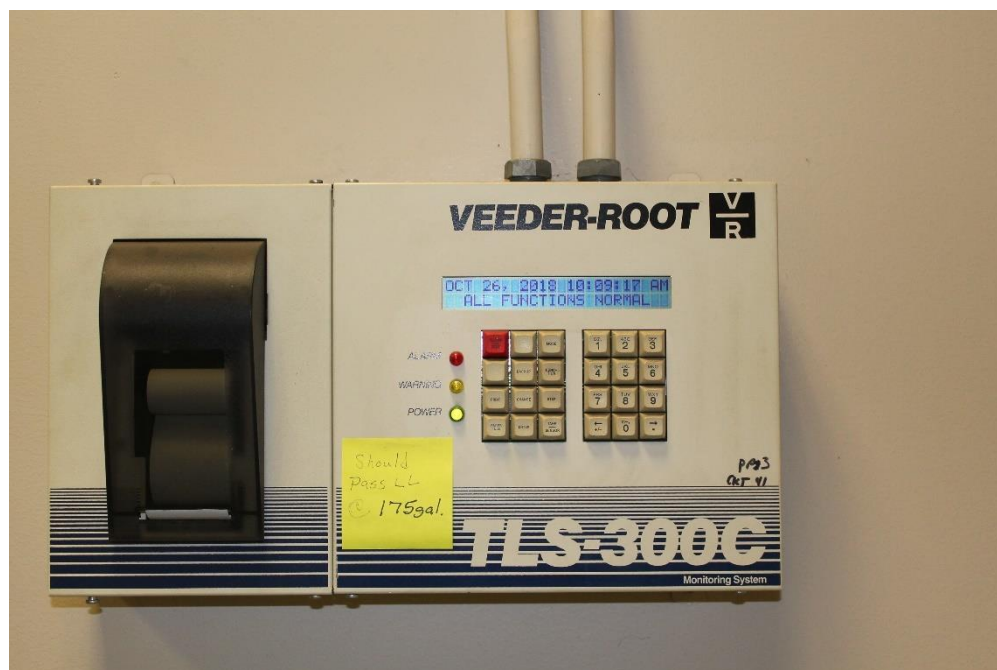
Figure 32. Monitoring system for an underground fuel storage tank. Photo Credit: Erik Ervin.
