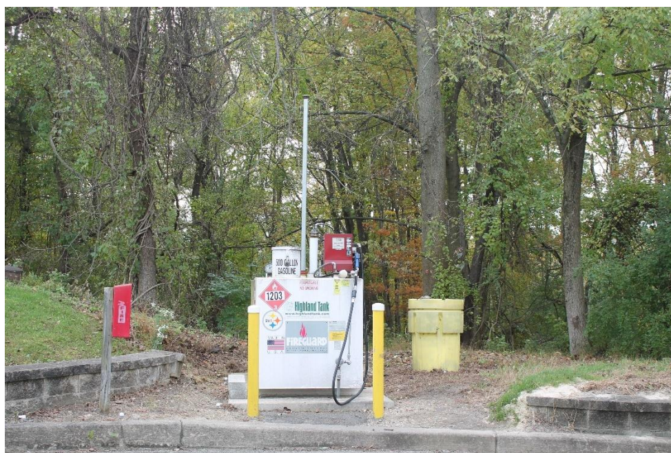
Figure 33. Fueling area includes fire suppression equipment and spill materials (yellow storage area). Photo Credit: Erik Ervin.
