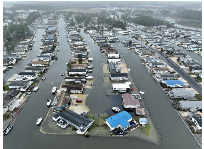
Figure 9. Flooded streets in Mariner's Cover during October 2025 nor'easter (Courtesy of Driscoll Drones)
