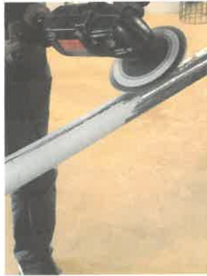
Stripping the paint from the pole
