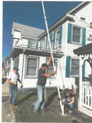
Reinstalling the flag pole
