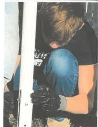
Tightening down the bolts
