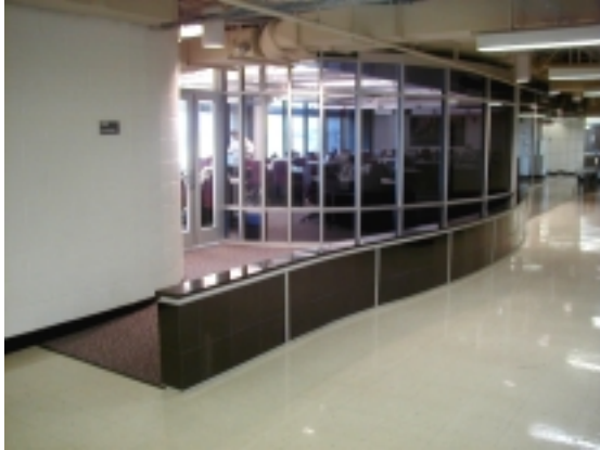
Figure 1: Tinted window wall between the learning center and the hall (used at both entrances)
