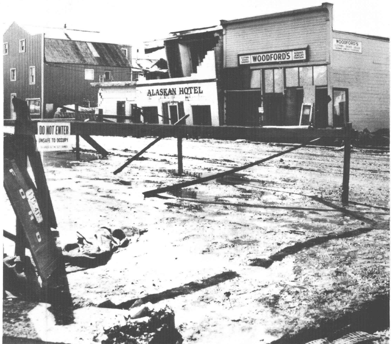
18.—Damage to the Alaskan Hotel on McKinley Street between Alaska Avenue and Broadway. The foundation of this building was intersected by four fissures. Photograph by T. L. Péwé.
