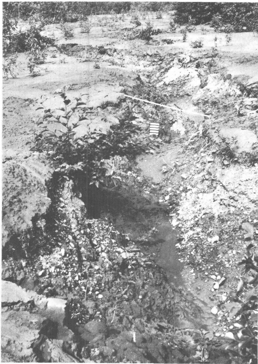
10.—Large longitudinal fissure. Surrounding area covered by ejected sand and silt. Carpenter's rule across fissure is 6 feet long; vertical scale below it is 1 foot high.
