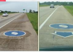
Figure 3-12: Hurricane evacuation route directional shoulder pavement markings
